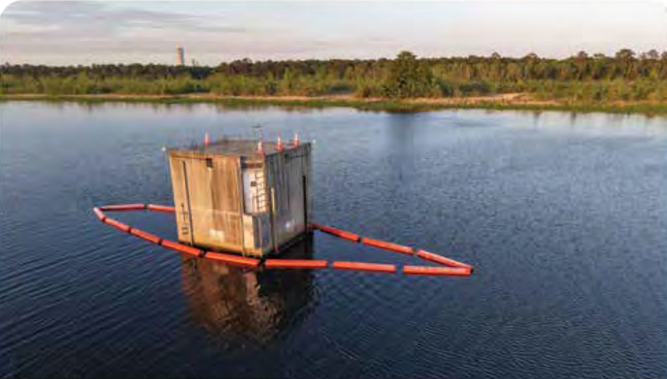
The CWS intake at Bushy Park Reservoir collects raw water and sends it to the Hanahan Water Treatment Plant.
